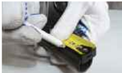
5. Mark on pipe the socket depth and a known value.
