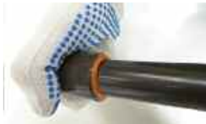
8. Push fitting straight home and hold for a few seconds.
