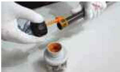
7. Apply solvent cement to fitting and pipe.
