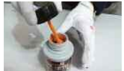
6. Stir solvent cement.
