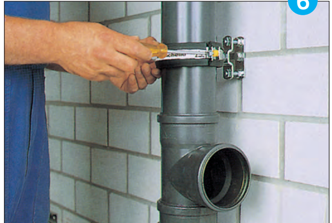
Assemble the support clip and secure the screws on the snap lock. A spacer prevents overtightening.
