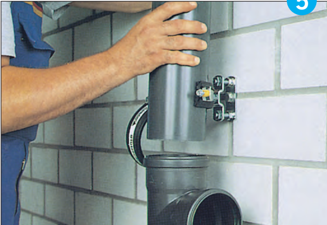
Open the snap lock of the support clip and insert the Friaphon pipe into the moulded fitting and clip fixer.
