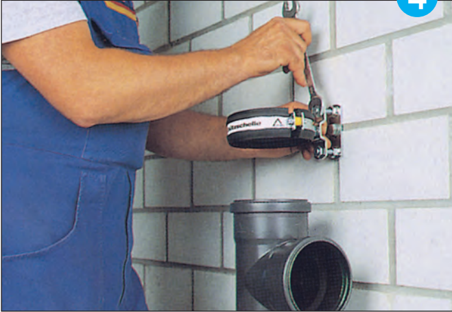
Fit the support clip to the wall attachment and tighten with a 17mm open ended spanner.
