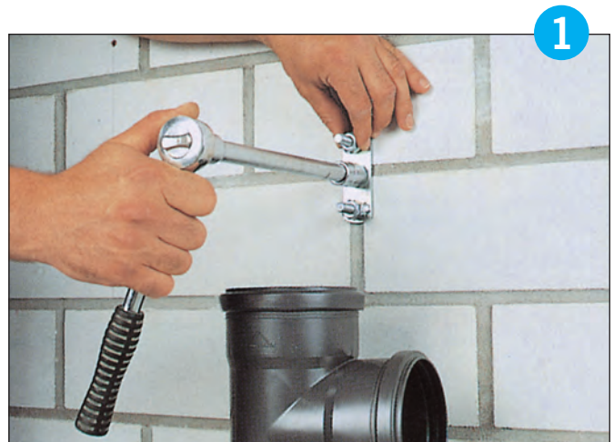
Mark, drill and fit the wall attachment.
