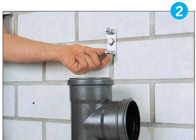
Adjusting the distance from the wall.
