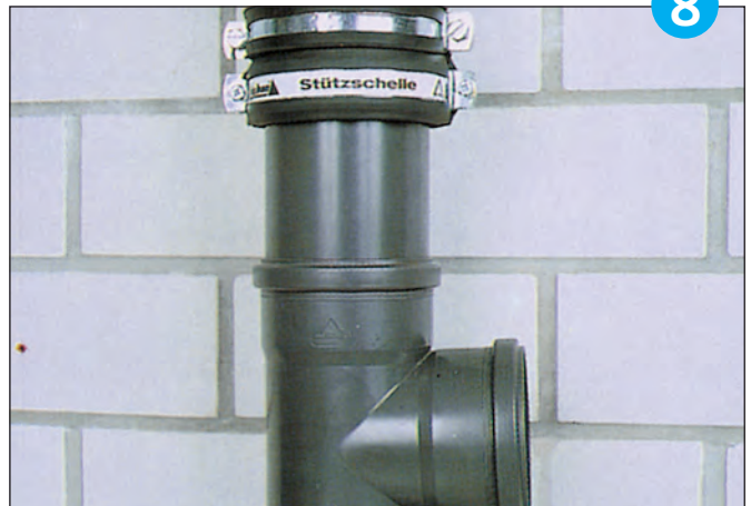
Finished assembly of the complete Friaphon support clip.
